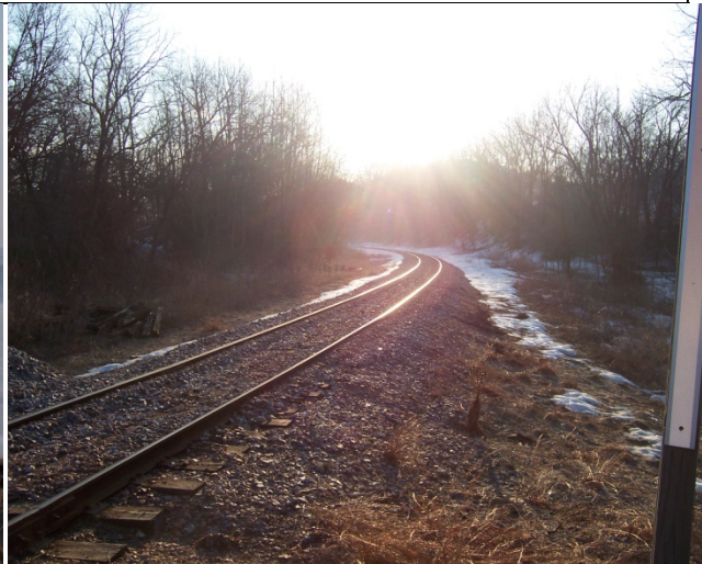
Figure 36 Section 7 & 12 Rail Corridor on Hwy 113 West View, Ferry & McCubbin Road
